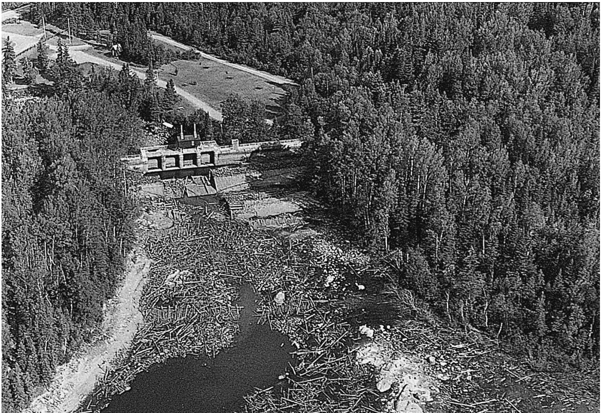
Fig. 5. Post-flood view of the concrete gravity dam that controlled the level of Lake Ha!Ha!. Lake basin is in the foreground. For scale, the four stoplog sluices within the dam are 4.56 m high.
