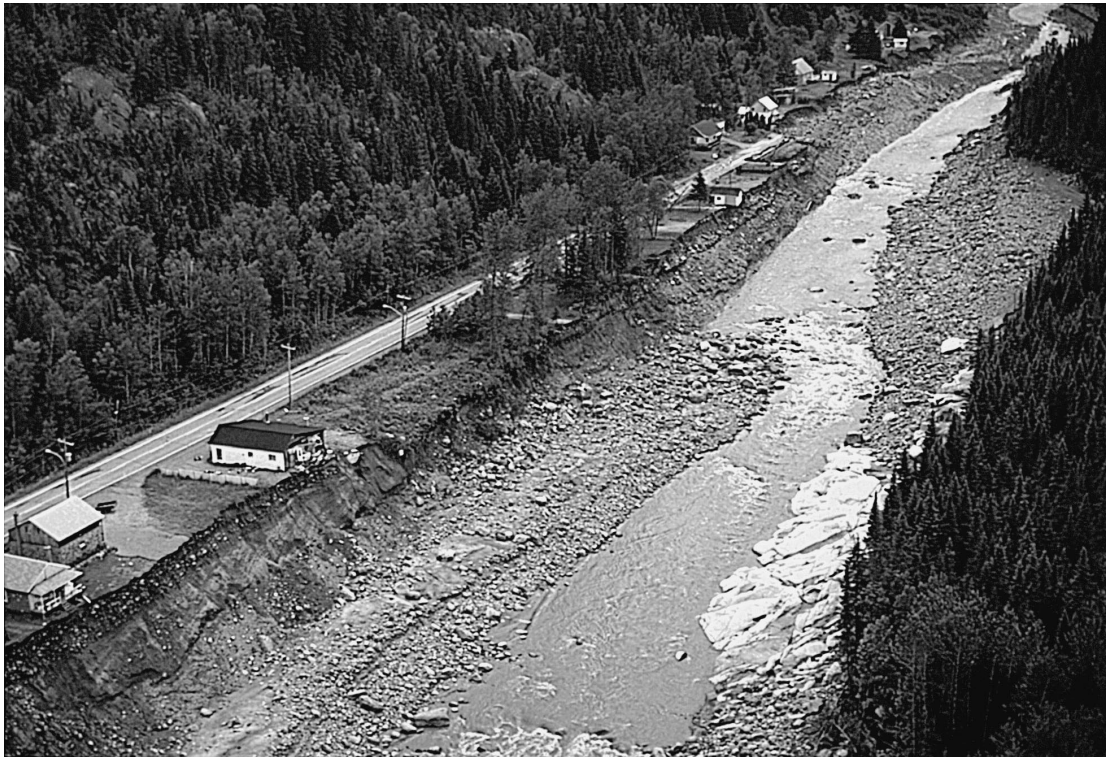
Fig. 15. The incised and widened channel, about 15 m deep, looking upstream from km 6. Exposed alluvium, diamicton and bedrock, and bouldery lag form the perimeter of the channel. Note the homes damaged by undermining along the right bank. Photograph taken on July 28, 1996 (GSC photograph 1997-42NN).
