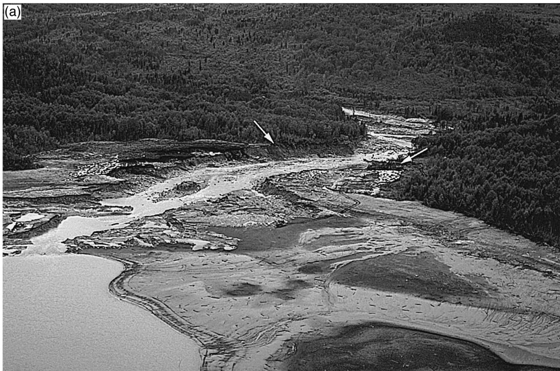
Fig. 7. The new outlet at the Lake Ha!Ha! reservoir that was eroded through the Cut-away dyke, (a) looking downstream from above the lake basin and (b) looking upstream into the drained lake basin. The outlet is about 130 m wide at the site of the dyke. In both pictures, visible locations of the remnant dyke are marked with arrows.
