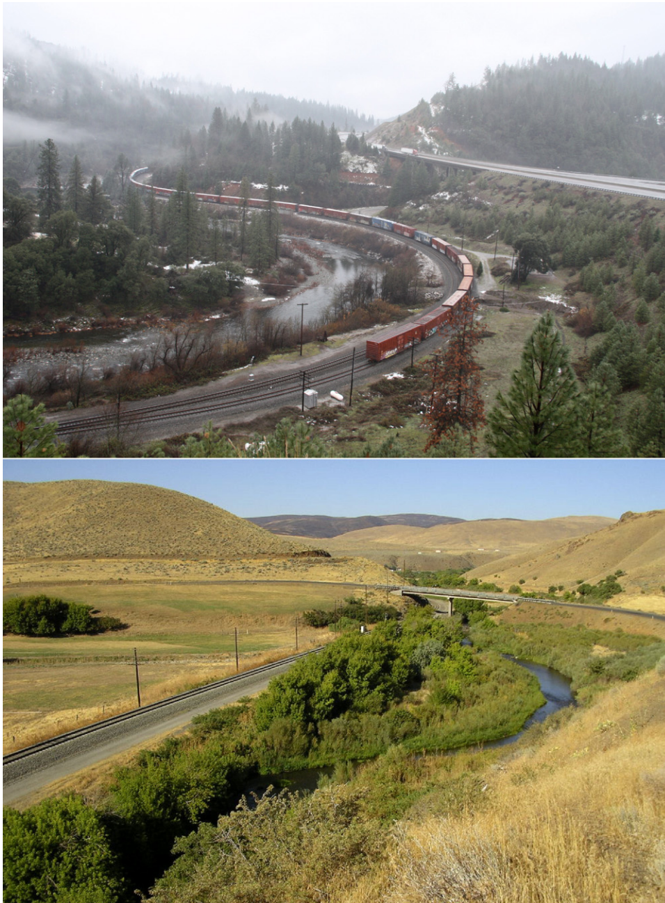
Fig. 1. Floodplain transportation lines. Top: Sacramento River, CA (photo courtesy of Kim Graves). Bottom: Umatilla River, OR. These features effectively act as lateral dams, disrupting lateral connectivity in the river landscape.
