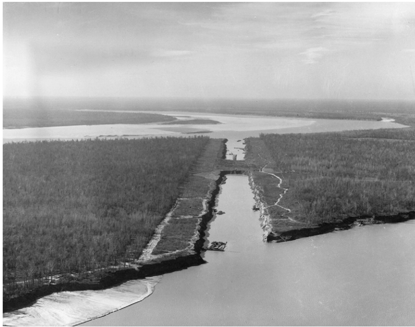
Fig. 10. Creation of pilot channel for meander neck cutoff at Jackson Pt.—Sunflower Cutoffs, looking upstream (photo: US-ACE).
