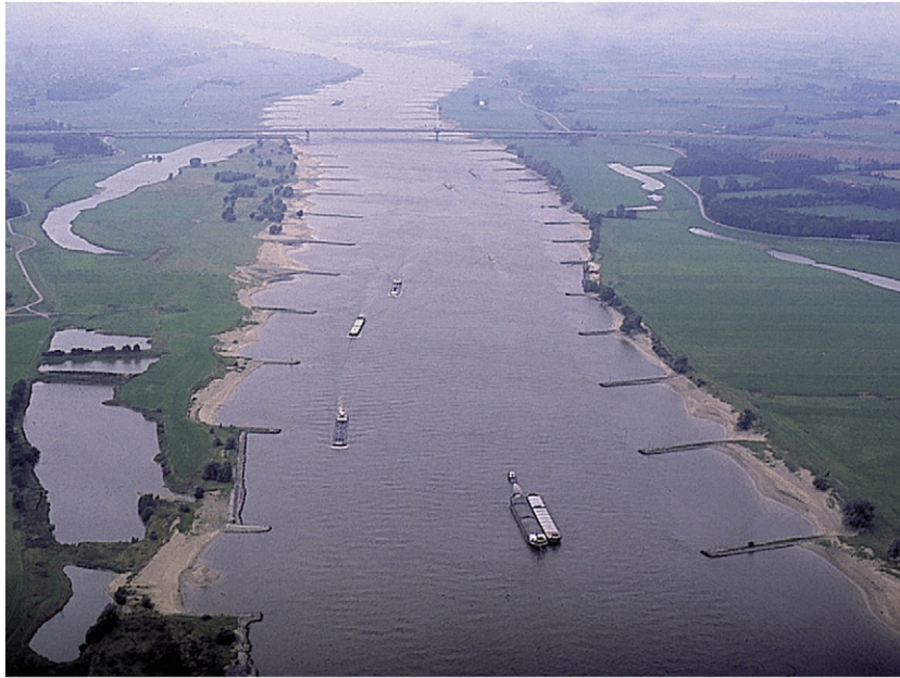
Fig. 25. The restrained Waal River. Photo showing river groynes and side channels within the embanked floodplain.
