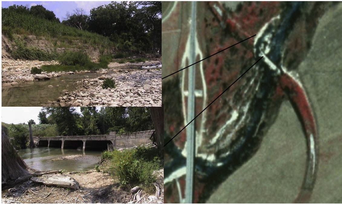
Fig. 9. The pre-existing low elevation road crossing was left in place after the new bridge was built. Wood and flood debris is trapped in the bridge openings and the channel is reworking avulsing around the old bridge. The new channel is shown in the photos on the left of the aerial photo.
