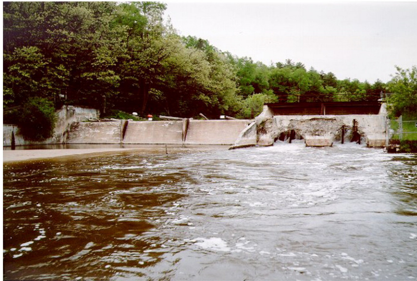
Fig. 1. Photograph of Stronach Dam in 2001, during gradual removal.
