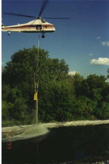
Application of Composite Aggregate Capping Material Using a Helicopter
