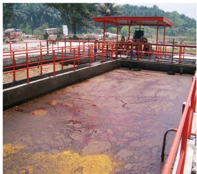
Picture 4: Effluent arising from the extraction of palm oil is temporarily stored in a cooling basin. Photograph: IFEU
