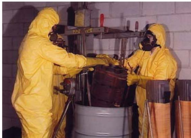
Packed piece-by-piece into steel drums, removed by elevator
