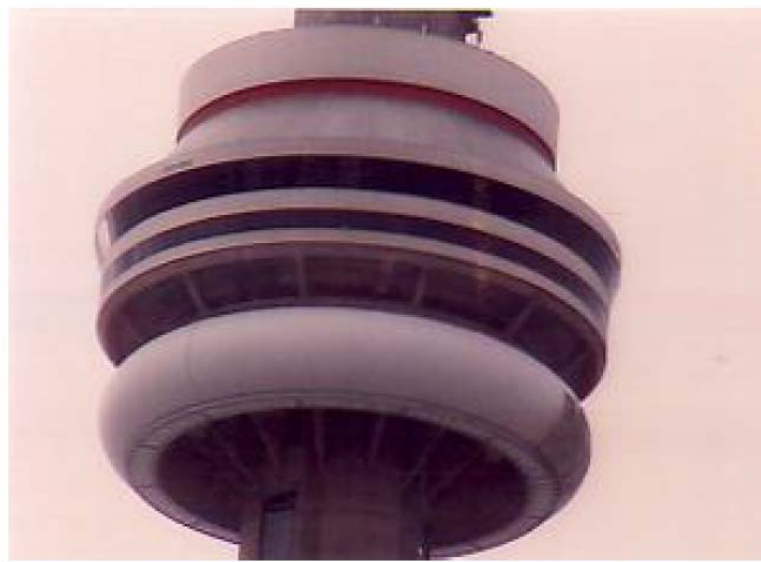
Transformer is located in viewing area, 342 m high
