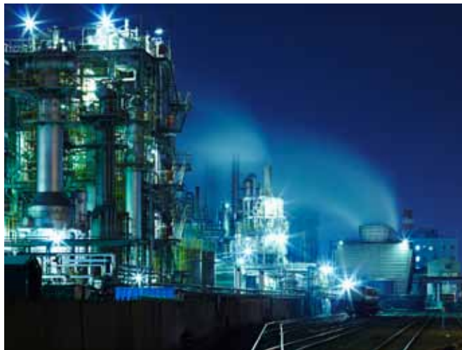
Large-scale chemical plant at night. © Tetsuo Morita/iStock
