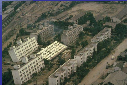
Buildings tilted due to soil liquefaction, 1964 earthquake, Japan.
