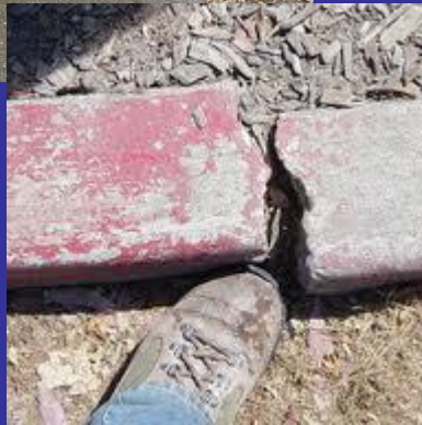
Berkeley, offset sidewalk
