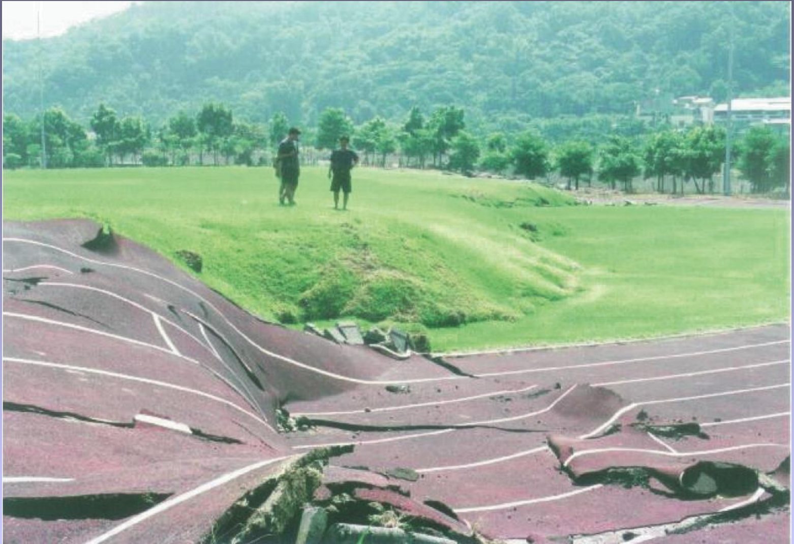
Chichi earthquake 1999, Taiwan
