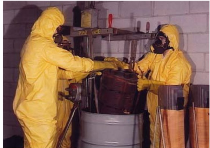
Packed piece-by-piece into steel drums, removed by elevator
