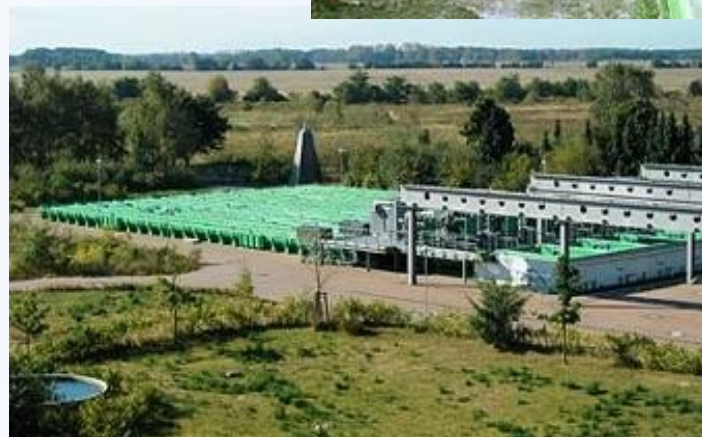
Figure 13. Artificial stream system of the Water, Soil and Air Hygiene Office, Marienfelde, Germany. Facility has been used to study the effects of sewage, nutrients, and detergents on stream ecosystem. Large building in the center is a pilot sewage treatment plant which contains automated sampling equipment. (Photo by P. D. Hansen.)
