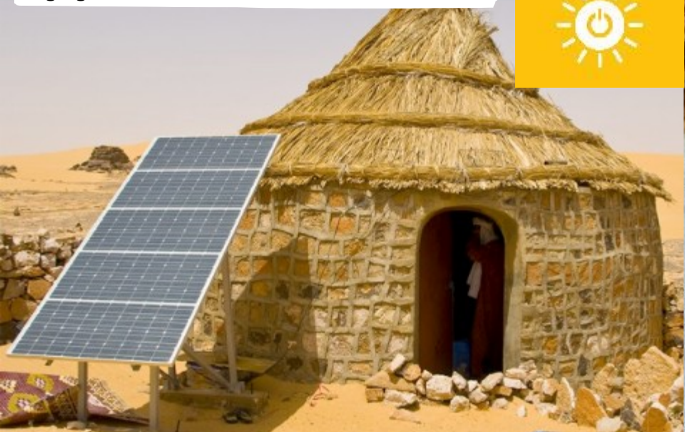
Darfur: Solar panels now provide the energy for a pump to provide 15 standpipes in the Khamsa Dagaig with water from the well.
