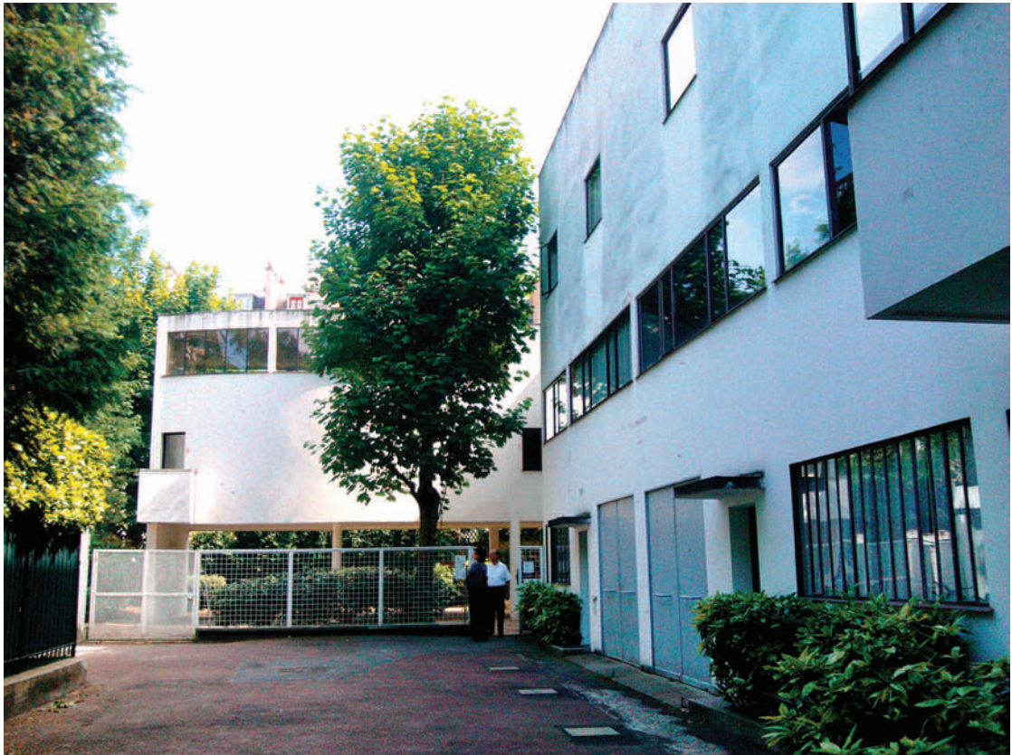
Figure 4.1 Villa La Roche, designed by Le Corbusier.
