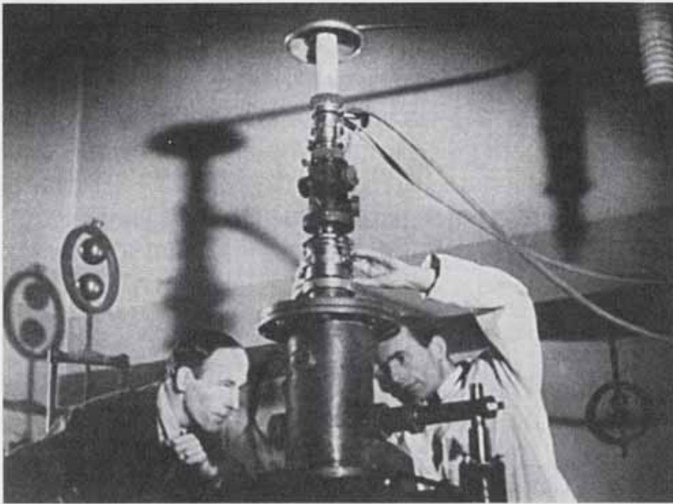
Figure 1.1. The electron microscope built by Ruska and Knoll in Berlin in the early 1930s.
