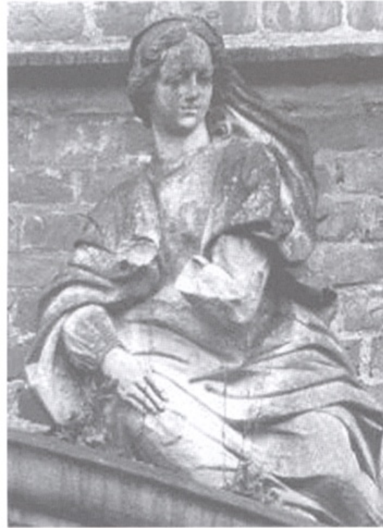
Figure 10.6. Sandstone figure over the portal of a castle, built in 1702, in Westphalia, Germany, photographed in 1908 (left) and in 1968 (right). The erosion of the figure is due to a combination of acid deposition and air pollution produced from the industrialized Ruhr region of Germany. Courtesy Herr Schmidt-Thomsen.
