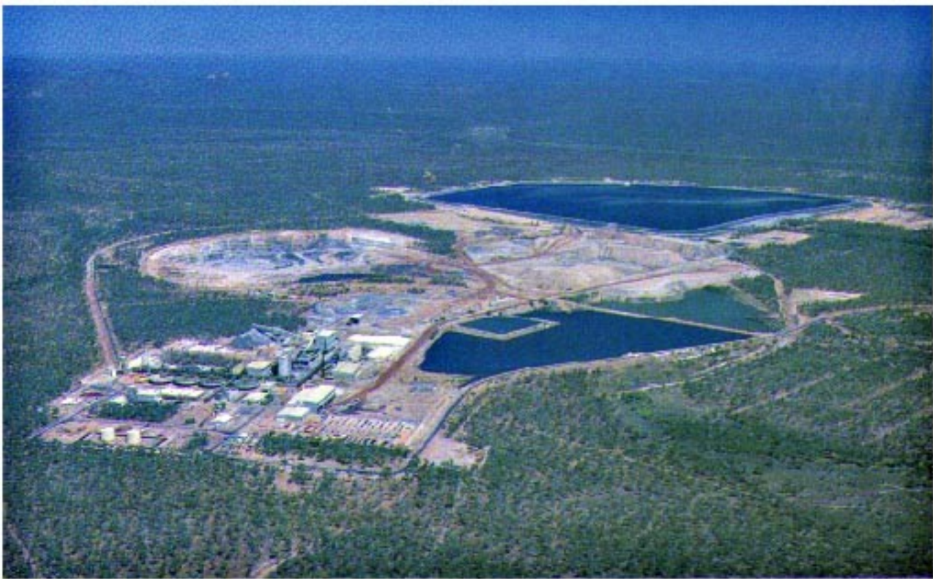
Aerial view of Ranger Mine and Plant
