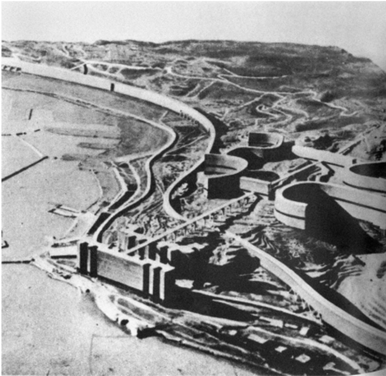
The 1933 rendering of Plan Obus for Algiers demonstrates Le Corbusier's superimposition of modern forms: the long arching roadway that includes housing-his viaduct city-connecting central Algiers to its suburbs and the curvilinear complex of housing in the heights that accesses the waterfront business district via an elevated highway bypassing the Casbah.
