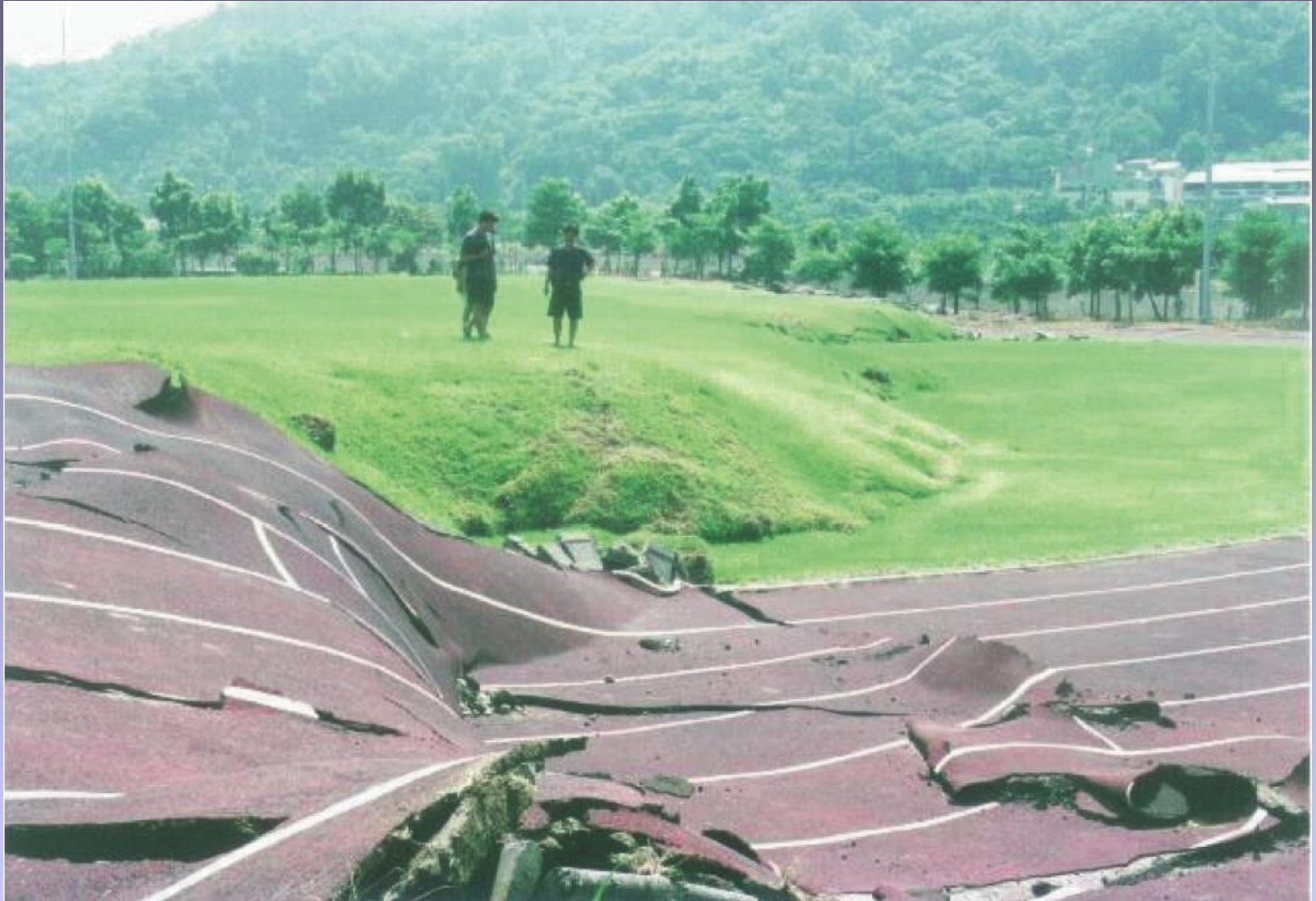
Chichi earthquake 1999, Taiwan
