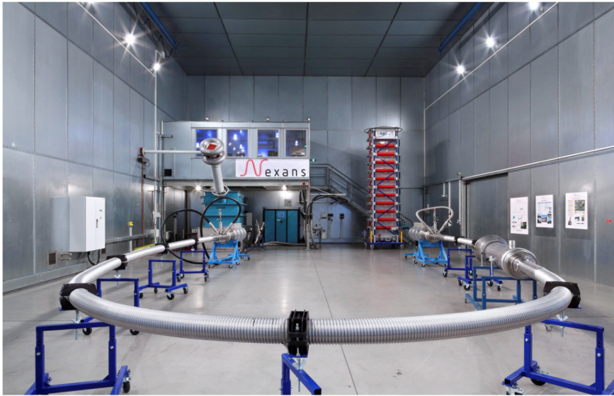
Fig. 5. Type test setup with prototype cable, terminations and joint.
