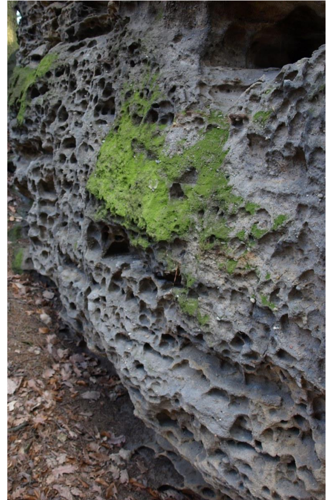
Weathering of a sandstone wall in Kokořínsk.
