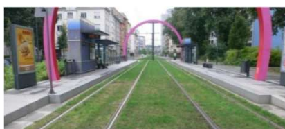
Green tram tracks (Mulhouse, France)
